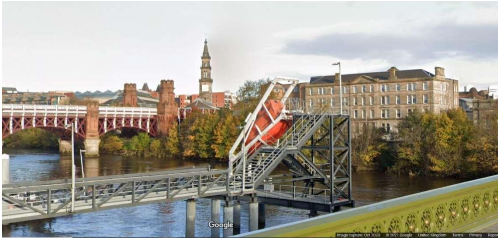
View from Albert Bridge. Google Streetview.
